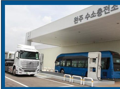
Jeonju, Korea Twin IC90 for Hyundai for commercial vehicle refueling Customer EMS; overall 7 HRS delivered to Korea in 2020
