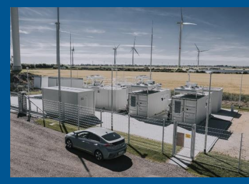
Schleswig-H., Germany IC90 & IC30 f. passenger car refueling and GH2 trailer fill at wind parks Customer GP Joule, 4 HRS in 2020 (3 HRS more in 2021)
